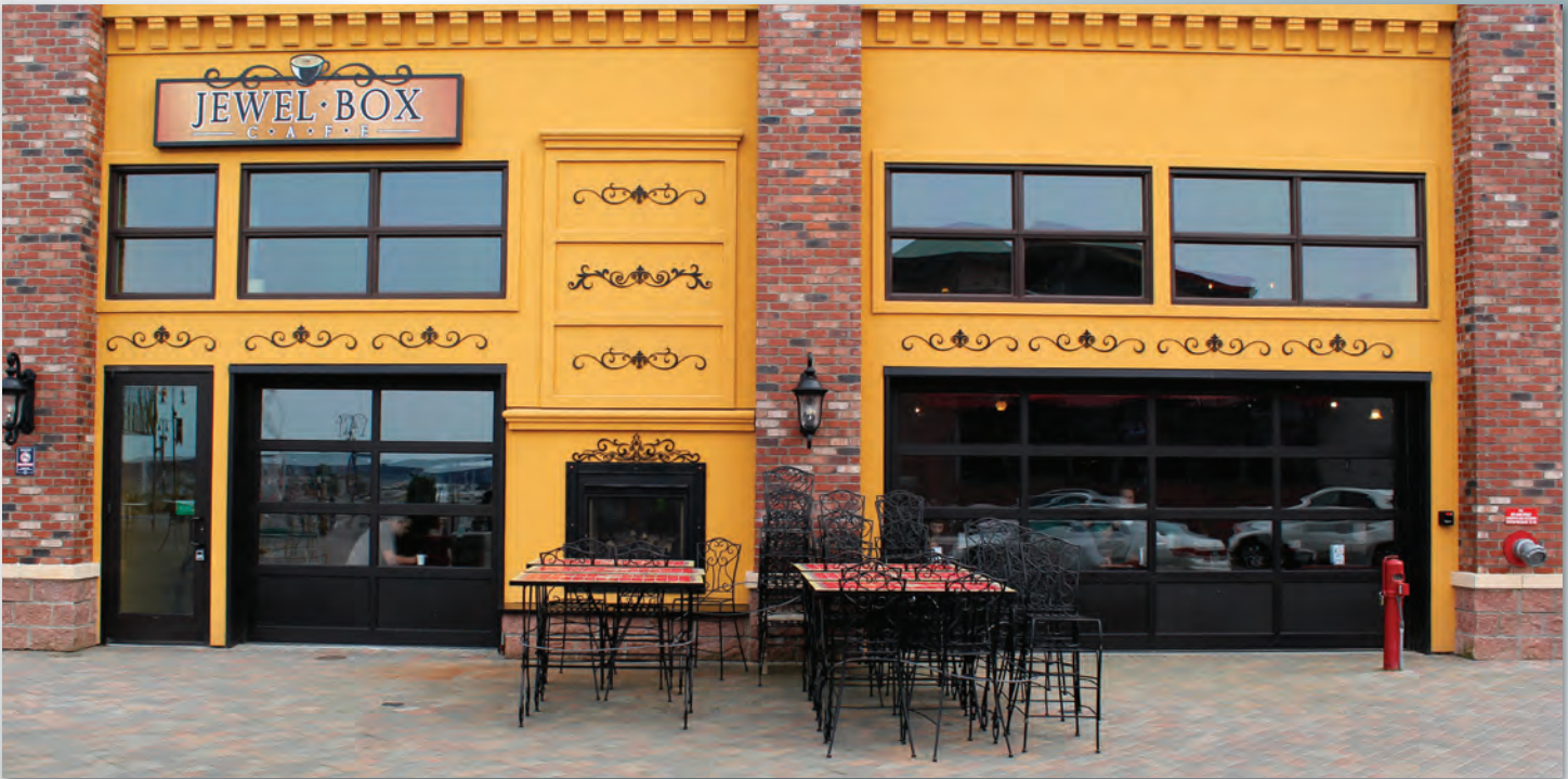
MC42-SC and MC44-DC, Dark Bronze Anodized with Clear Tempered Glass in upper sections and Solid Aluminum Panels in the bottom sections.
